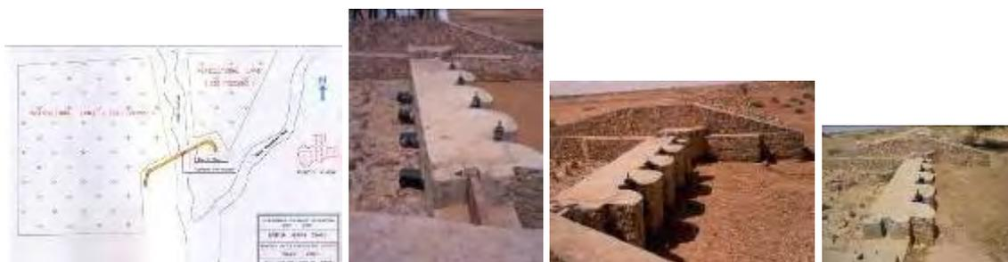
Original designs from Azagarfa dam, dam in use, dam post-construction and dam now, silted up (planned by village development council and designed by PAC)
